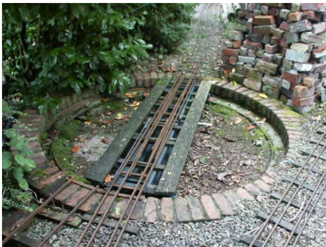
The turntable – note the additional steelwork to switch sides when turning 5" and 3-1/2" gauge locos. The spur to the carriage shed is to the right and the embryo 'loading line' to load or offload to a trailer is to the left.
